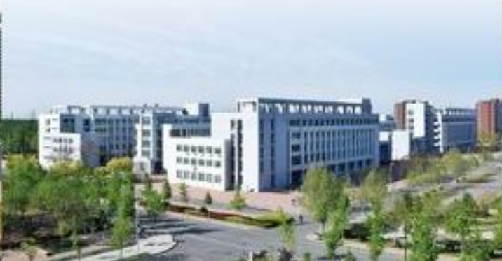
中国民航大学项目 Municipal Pipe Network of Civil Aviation University of China
